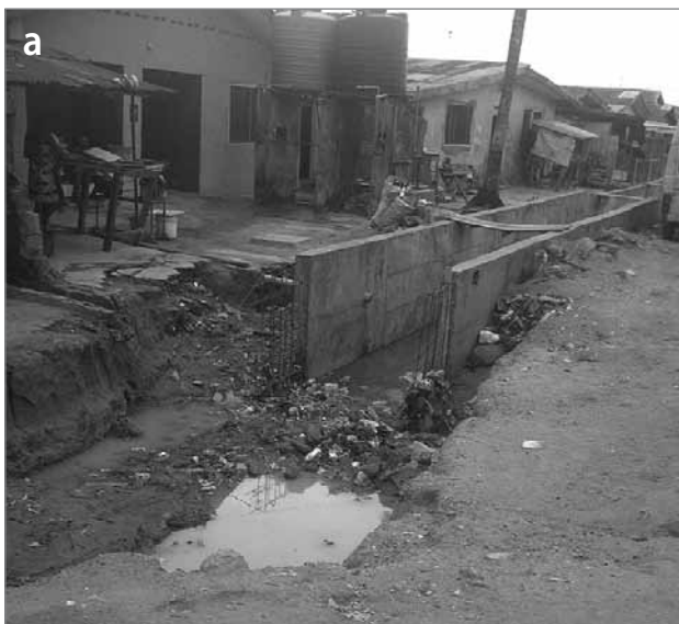
Figure 4: Storm-water drainage in Ayobo (adapted from Opoko, 2013).
