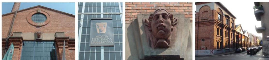
Figure 6: The Old Ljubljana Electricity Power Station (source: Pichler-Milanovič & Foški, 2014).
